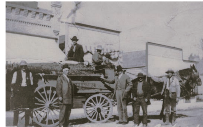
First load of water pipe: "Sherriff DeVilbiss and William Dinkel stand near the back wheel of the first wagonload of water pipe arriving in Carbondale in 1910." DeBeque Collection photo
